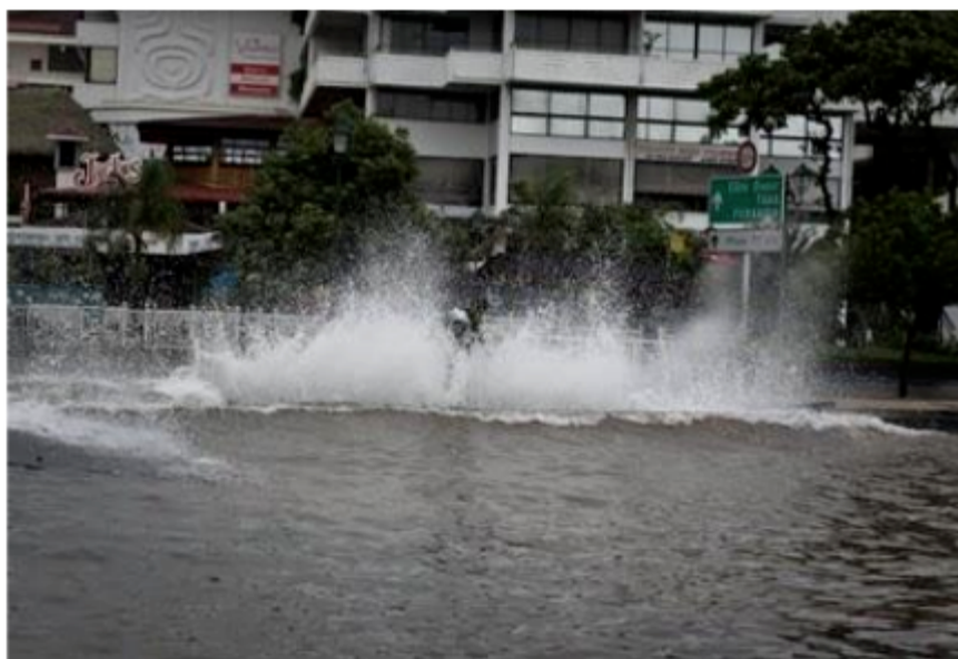
Figure 10 – Inundation of the circular coastal road in Papeete during cyclone Oli (2010).
