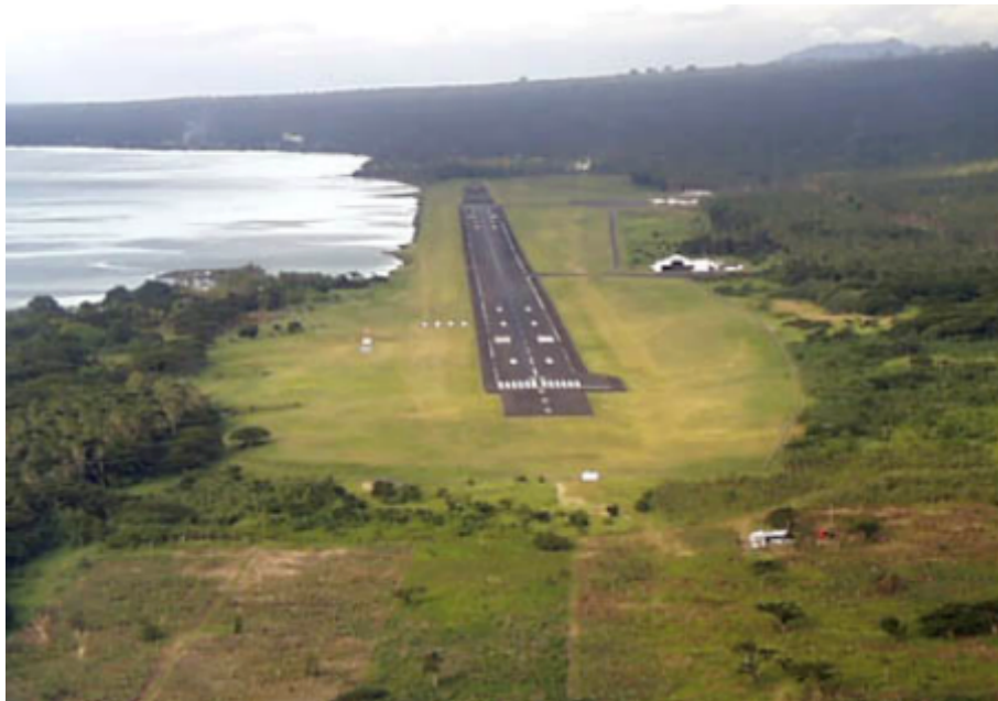
Figure 8 – Coastal landing strip in Samoa. Source: Baker and Week 2012.
